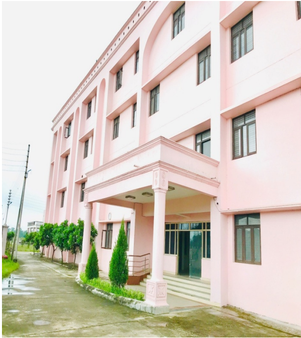
Exterior View of Boys Hostel
